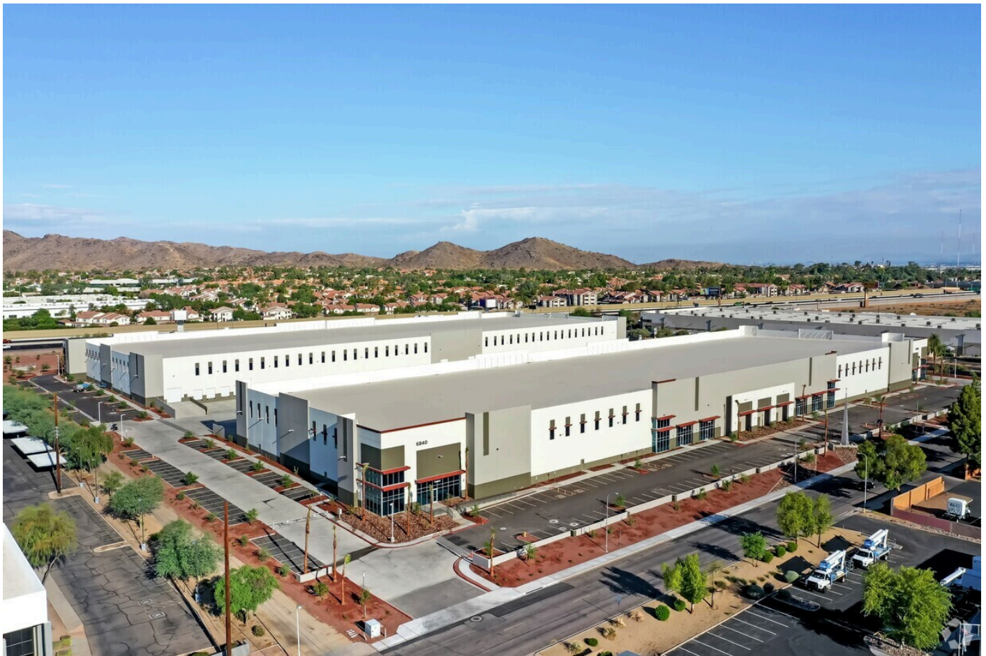
ViaWest Group redeveloped a vacated former office complex into what is now Sight Logistics Park in Tempe, Arizona. (CoStar)
